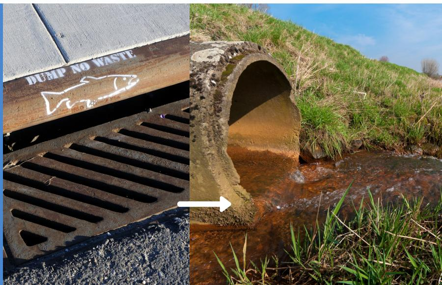
Stormwater runoff is simply rainwater that does not soak into the ground, but runs off hard surfaces like paved streets, parking lots, sidewalks and rooftops. As stormwater travels, it can pick up pollutants along the way. This stormwater pollution enters our waterways and can be detrimental to water quality and aquatic life. The storm drainage system in Monroe is a network of storm drain inlets and underground pipes that carry stormwater from our streets directly to our streams.
