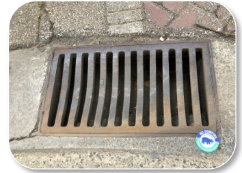
Drainage systems are designed to reduce localized flooding. Storm drains discharge to local waterways without treatment .
