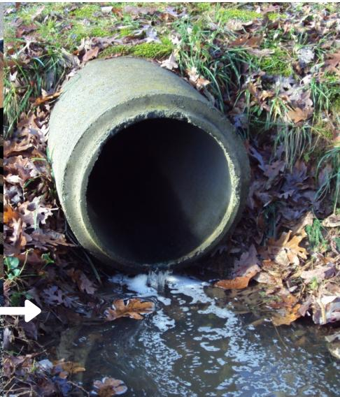
Storm drainage systems are designed to prevent flooding by collecting stormwater when it rains. This stormwater flows over surfaces, picks up pollutants, and eventually discharges into lakes, streams, and rivers. Unfortunately, there is no treatment process in the storm drain system to filter out pollutants before they reach downstream waters.
