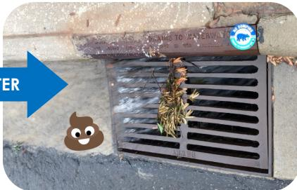
Since our **storm drainage system is not connected** to any type of treatment plant, these pollutants are discharged in the closest creek, stream, river or lake.
