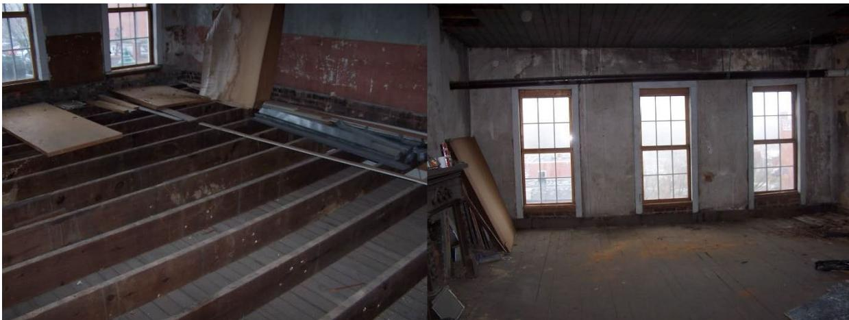
The roof system consists of single slope wood trusses bearing in the center and exterior masonry walls. Masonry walls at the perimeter and center of the building extend above the wood roof trusses forming a flat parapet at the building front and two sides. Roof decking is wood with a membrane roof system over top.
