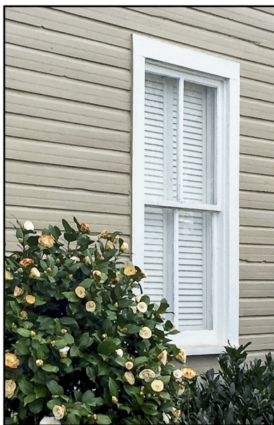
Wood windows, when properly maintained, enhance both the aesthetic quality and energy efficiency of a home. Operable windows allow for the capture of cooling breezes, while historic wood windows paired with storm windows offer an equivalent increase in energy efficiency to contemporary double-glazed windows.
