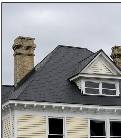
Significantly deteriorated or damaged metal shingle roofs can be replaced with compatible new metal shingles. Above, new pressed metal shingles were fabricated to match the dimensions and profile of the original metal shingles.
