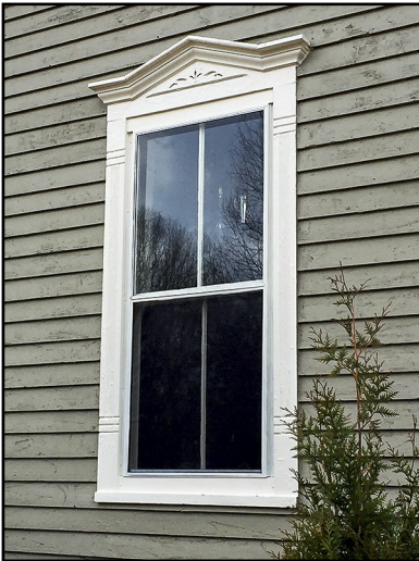
The installation of storm windows and doors is one of the most common ways to increase the efficiency of historic windows and doors.
