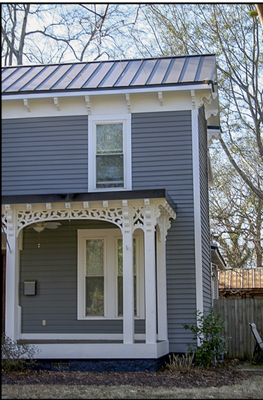
Modern metal roofing is commercially available for roofs deteriorated beyond repair. However, care should be taken to select a product with a ridge profile that is comparable to a true standing-seam roof.
