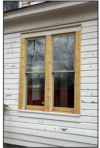
Replacement windows should match the originals in material, dimension, pane configuration, and detail.
