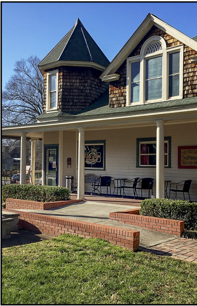
Commercial buildings in the historic district must have wheelchair access to be ADA compliant. This is often achieved through the installation of brick or concrete ramps.
