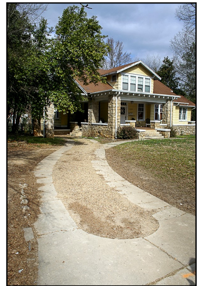
Paving strips, or ribbon driveways, have less impervious surface area and thus, reduce runoff from the site.
