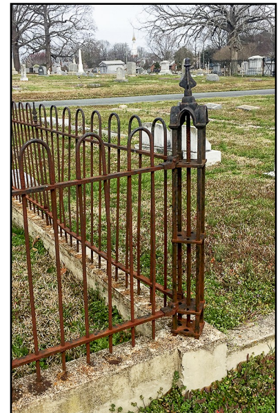
Wrought iron fences are common in the district and the Monroe Cemetery. All require protective coatings to minimize oxidation and subsequent corrosion.
