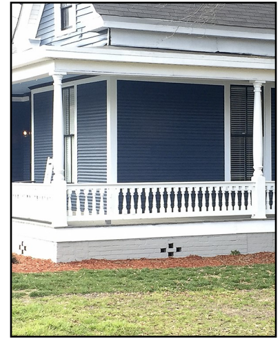
Brick and concrete are used throughout the district for building foundations, eliminating contact between the ground and wooden elements of buildings. Foundation vents allow for air circulation beneath buildings.
