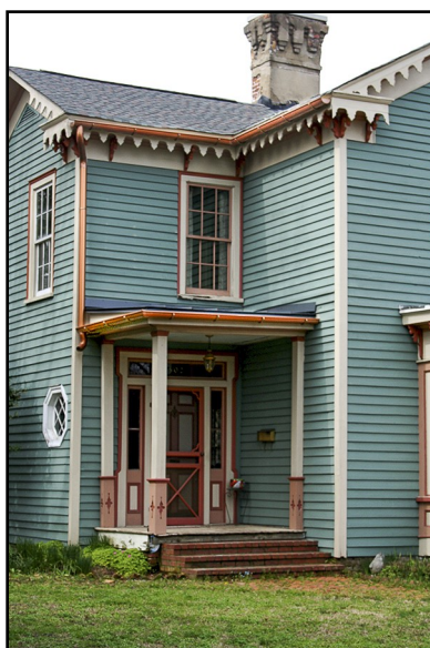
Copper, which develops a patina in response to atmospheric corrosion, is an ideal material choice for gutters and downspouts (above), due to its long-term durability without painting. Alternatively, aluminum with a factory-applied color finish is a more cost effective metal for the same application.
