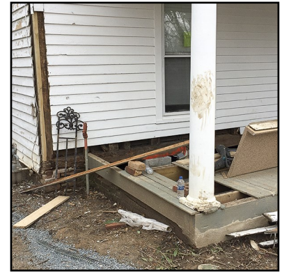
Above, deteriorated sections of wooden elements including clapboards, corner-boards, porch flooring, and a porch column base were replaced in kind. The image below shows the completed repairs freshly painted.
