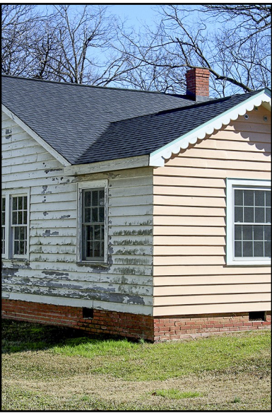
The removal of all loose and peeling paint is necessary to ensure that the new paint will adhere fully.
