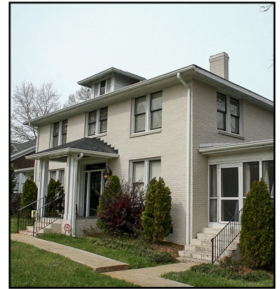
The inclusion of handrails improves access for all occupants. The railing to this side porch was manufactured to match existing front porch railings.
