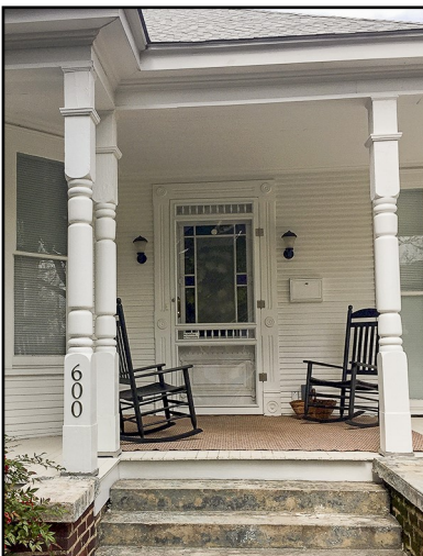
Made from an original screened door, this storm door features a low profile that allows for a clear view of the colored glass panes in the historic door.
