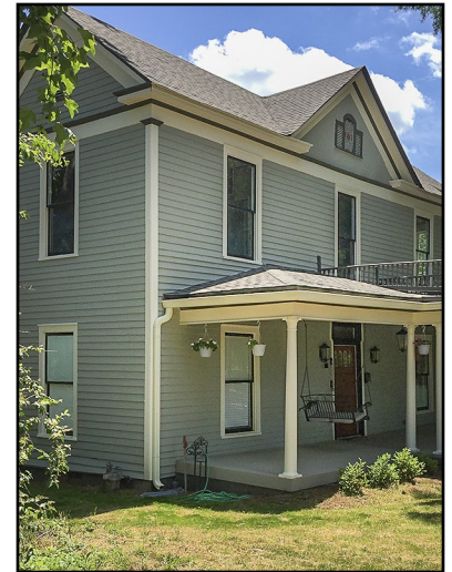
Above, deteriorated sections of wooden elements including clapboards, corner-boards, porch flooring, and a porch column base were replaced in kind. The image below shows the completed repairs freshly painted.
