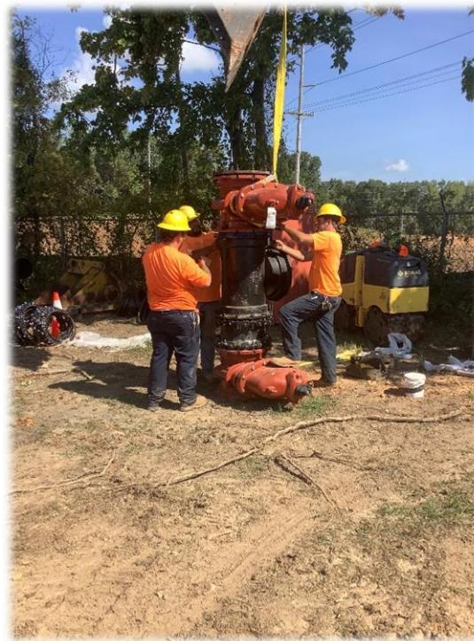
Our Construction crew is laying 16" Ductile Iron Pipe towards the Patton Elevated Storage Tank
