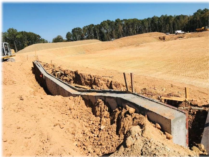
Topsoil is spread as an underlayment for the liner installation:
