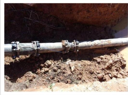
Shown: Creek crossing construction and new water main with tracer wire for future electronic location of the main. Also shown, Equipment Operator III Manny Carrillo injecting a chlorine solution into the new main. Every new water main must undergo bacteriological disinfection and pass rigorous laboratory testing before serving water to Monroe customers.
